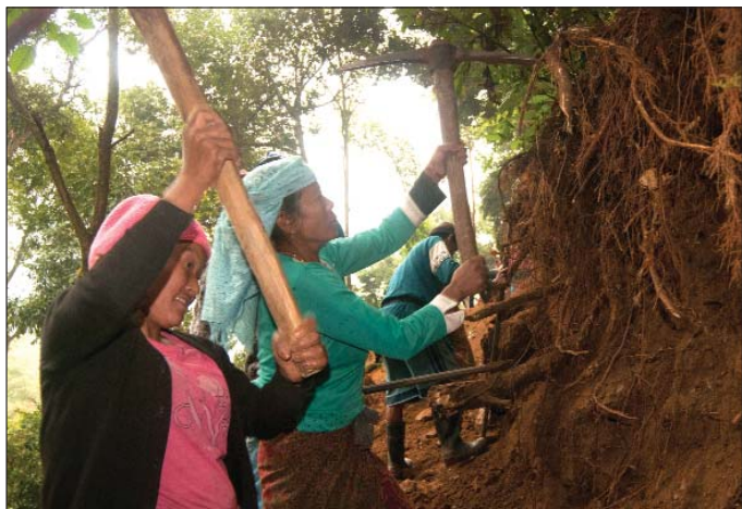
Women participating in rural road construction (Jhyaunpokhari, Bhojpur)
