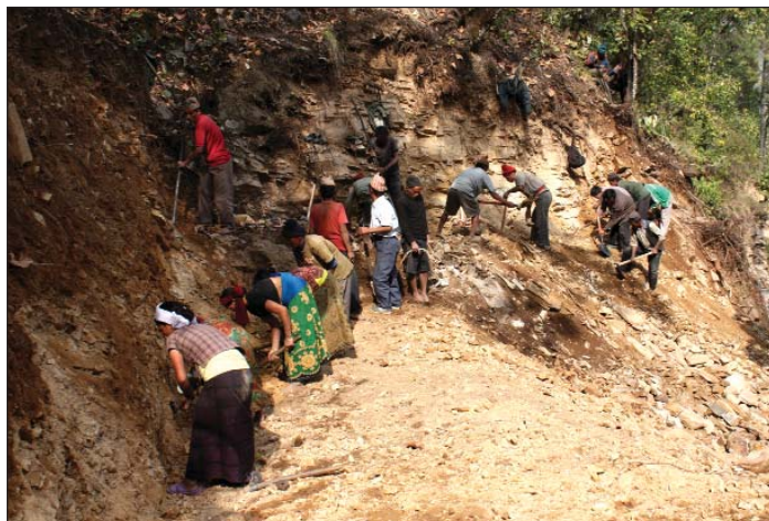
Women participation in agriculture road construction, Dailekh District
