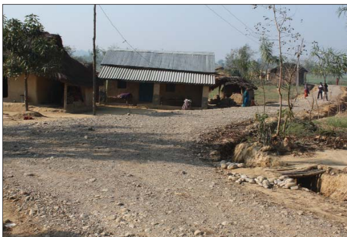
Road constructed in a remote village in Banke district
